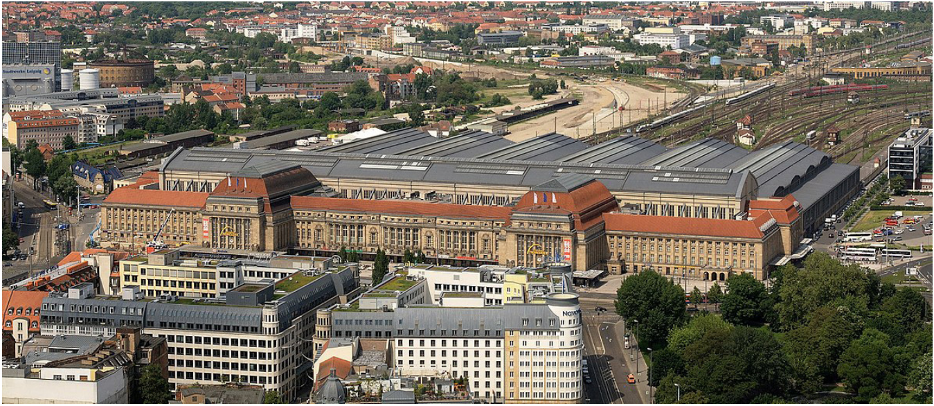
Figure 3. Leipzig Main Train Station. (Source: Wikimedia Commons).
